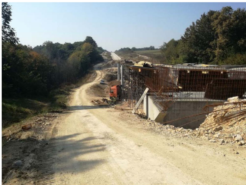
View of ongoing construction works on Brčko Bypass, Bosnia and Herzegovina.
