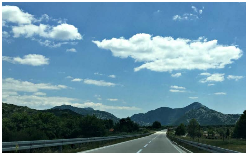
Landscape and infrastructure on the route from Vilusi to Herceg Novi, Montenegro.
