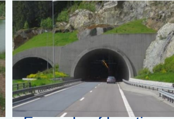
Example of location of safety barriers at tunnel portals
