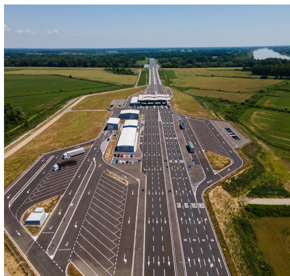
Svilaj cross-border bridge on Corridor Vc, © JP Autoceste FBiH
